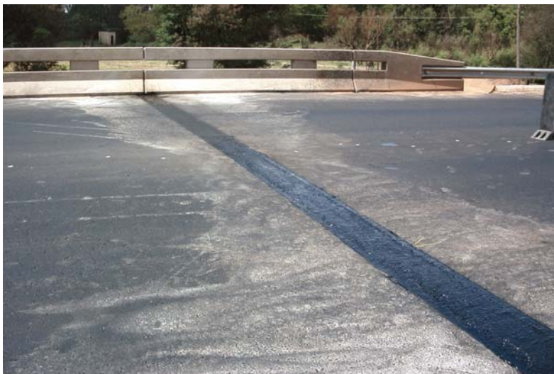
Finished Thormajoint® bridge deck expansion joint.
