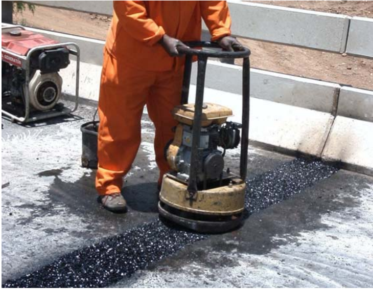
The top layer is compacted level with the adjacent road surface.
